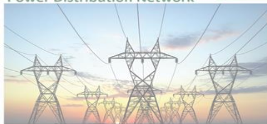
Power Distribution Network
